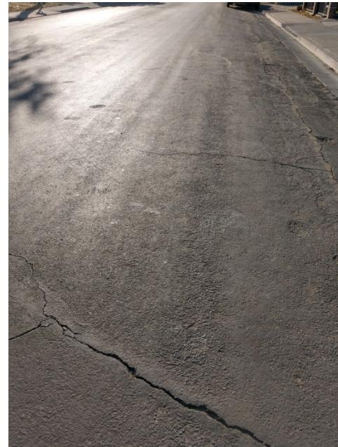
**Figure 15:** Fog sealed and striped road rated at 81 PCI (satisfactory condition) located on F Street in Los Banos.
